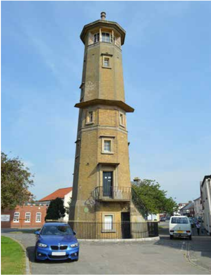
ABOVE: The high, rear light of a pair of leading lights established in the 17th century at Harwich. A low light was located on the beach some 200 m distant.
