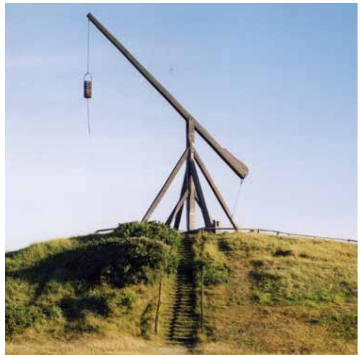
ABOVE: A replica of a swape light or vippefyr that was used at Spurn Head (1674). This one is at Skagen in Denmark, here on a hill rather than a stone tower.
