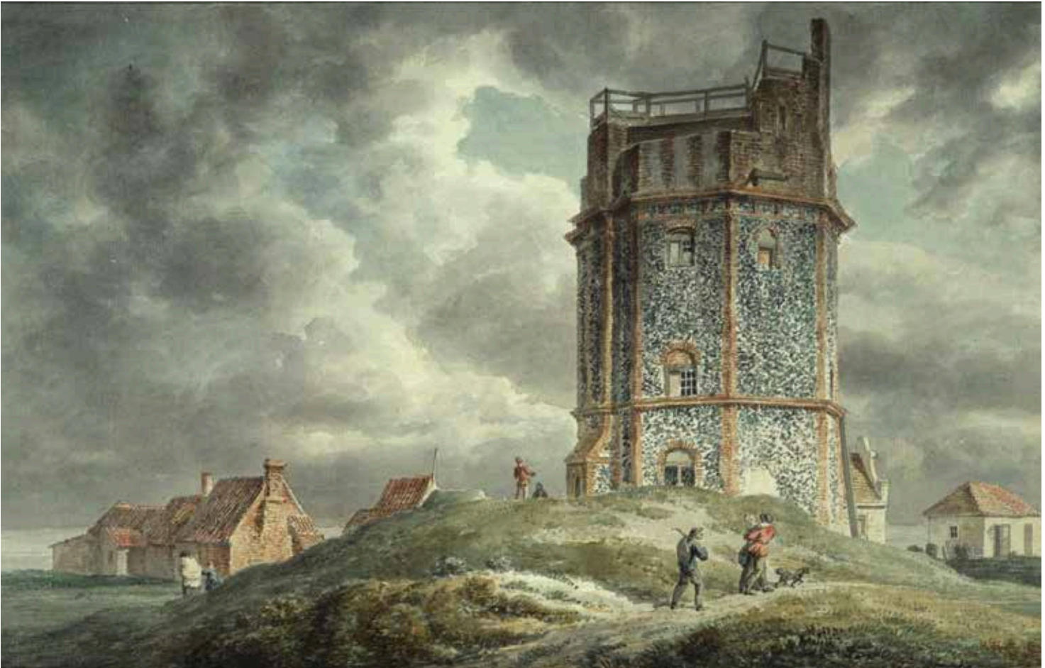
ABOVE: A painting of the North Foreland lighthouse in its form from 1691 to 1793. The tower is of stone and a coal-filled chaffer was kept burning throughout the hours of darkness.
